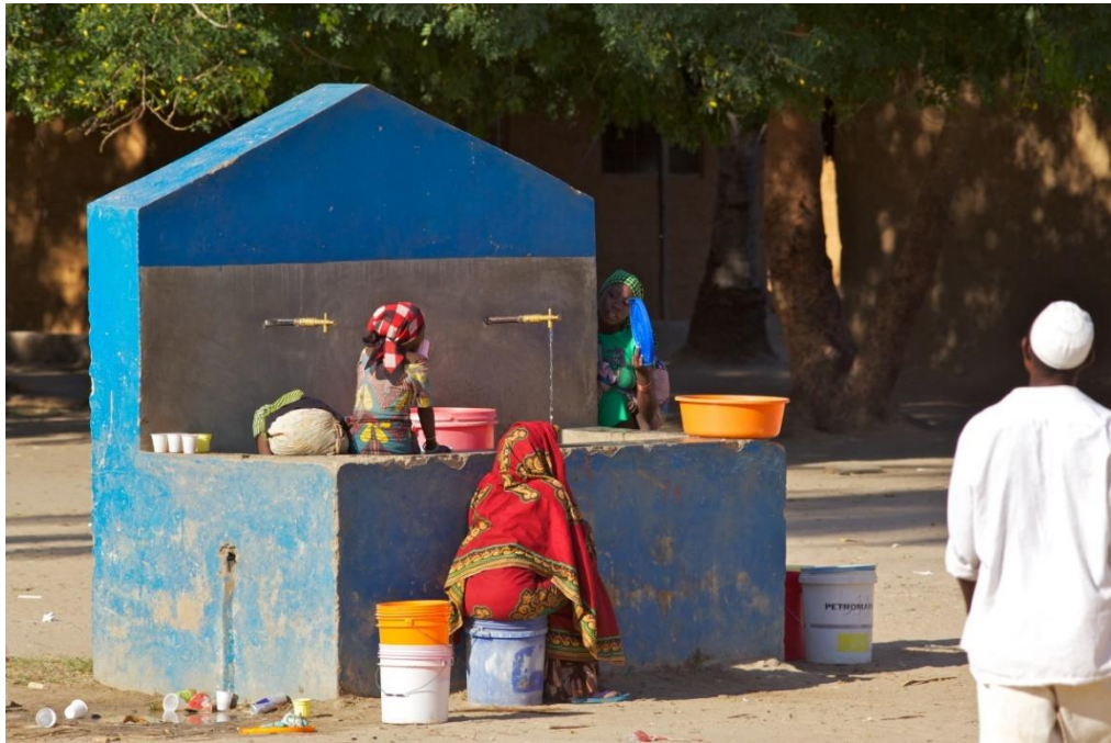
Communal water supply
