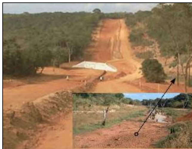
Figure 4.19: Dry road culverts on route from Palma to Olumbe turn-off. (Left) culvert at section D
