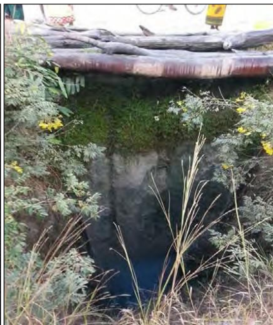
Figure 23: Deep hand-dug well with the water table at ~5.6m near the village with centralized water
